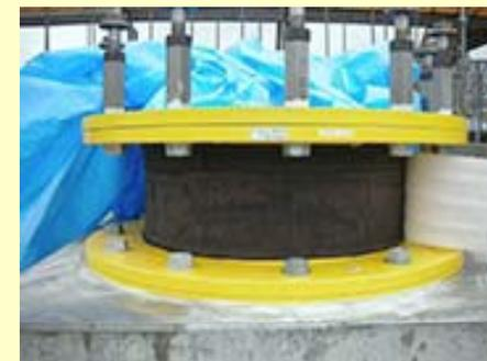
Base isolation system (laminated rubber isolater)
